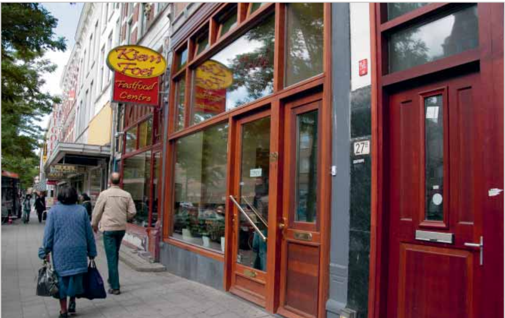
Improvement of plinth facades
