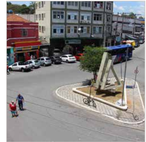
Example of roads (after), São Paulo, Brazil
