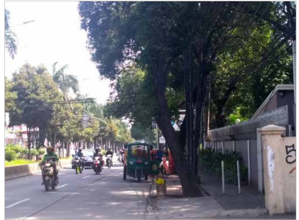
Walkway condition in front of a school along an arterial road
