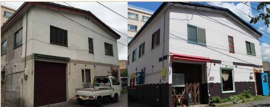
A building on the Green Street before (left) and after (right).
