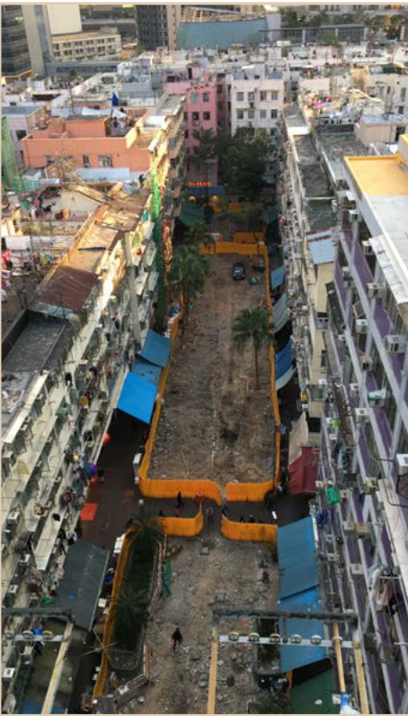
Construction site of Yi Pei Square Playground, Tsuen Wan. Going beyond conceptual ideation, the aim is to transform the micro-park designs into reality.
