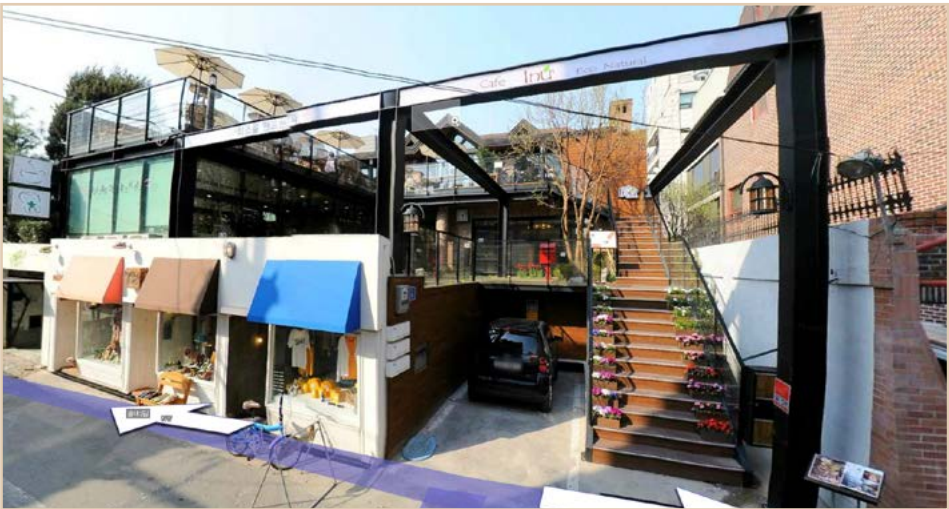
A property in Hongdae before renovations (top; 2009) and after (bottom; 2011).
