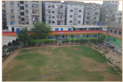
DCTO School football court under construction
